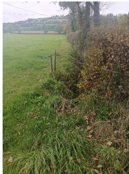
Plate 11-8: Land Drain IDB6
