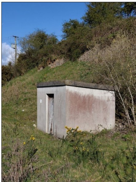
Plate 11-15: An example of structures that make up the buildings and artificial structures (BL3) within the site
